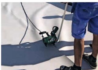
Suitable for flat and steep/pitched roofs due to clamping system. For perfect welding seams on any underground.
